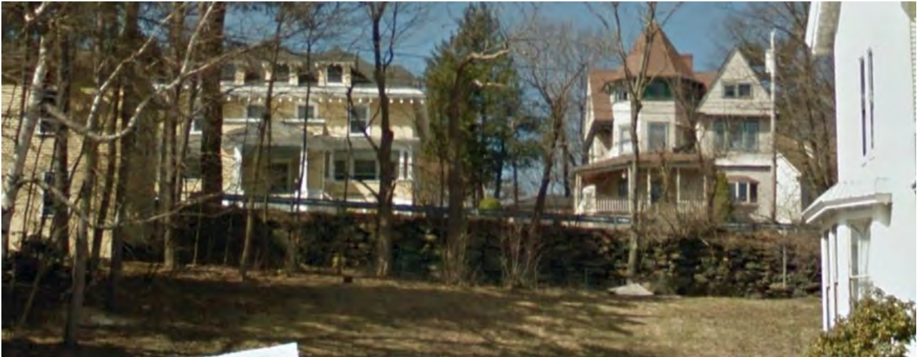
*Opposite 32 Beacon Ave – This wall was constructed by the City sometime after May 6, 1912 after approval of a petition to the City for a bank wall on the east side of Beacon St from Western Av to the angle in the street. *In FY15 CIP
