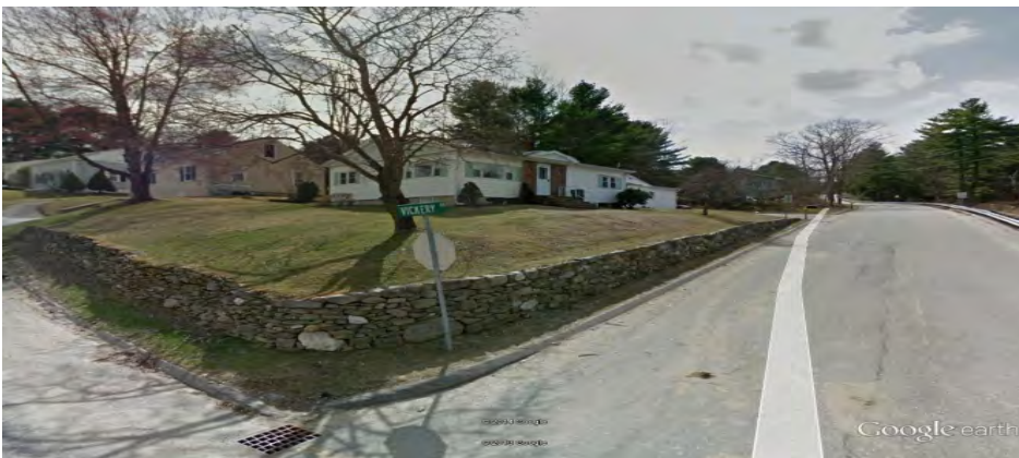
Vickery Road, starting at Riverside Drive – Dry stack stone wall repaired in 2004.
