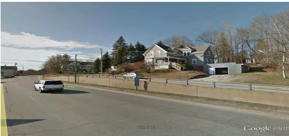
Washington Avenue, between Minot Ave. and Jefferston St. – Concrete wall constructed in 1957.
