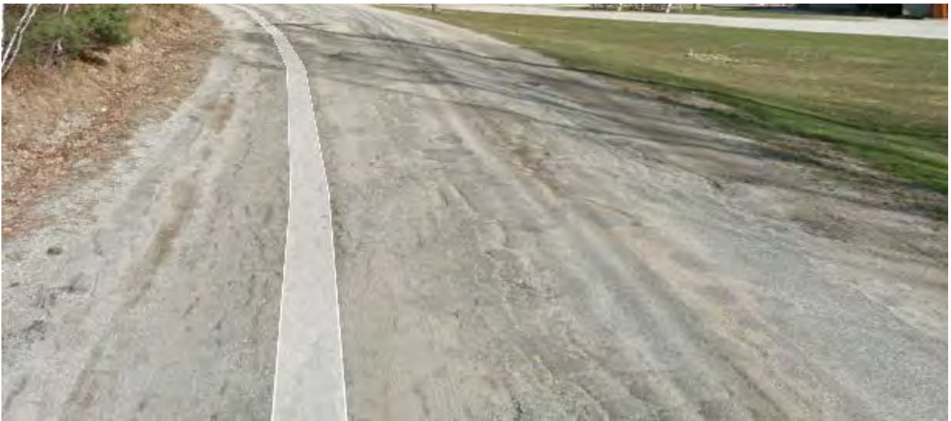
Summer Street (3000 lf) from Park to Mount Auburn – The roadway has a PCI rating of 37.58. The roadway will be converted to a one way in-bound with a turn-around outbound after the last driveway. The estimate for the reconstruction is $400,000.
