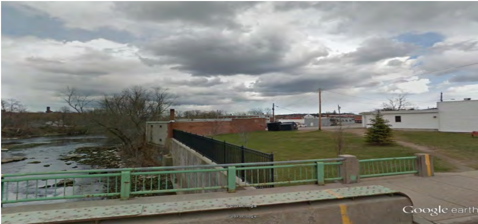
South Main Street, downstream side of Main Street bridge over the Little Androscoggin – Replaced a stone wall and was constructed in 1996.
