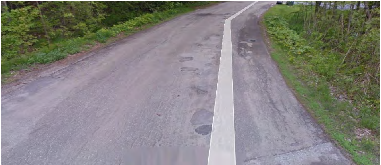
Valview Drive (7500 lf) from Garfield to dead end – The roadway has a PCI rating of 41.08. The estimate for the reconstruction is $1.25 million.
