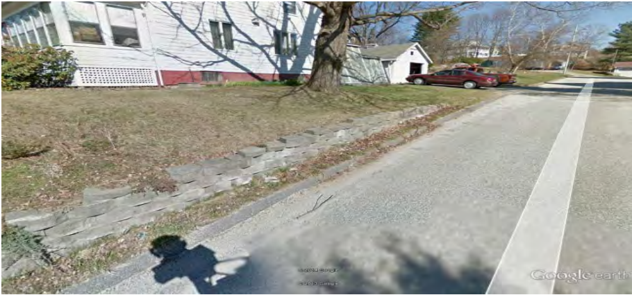
North Side of Atwood Street at 18 Poland Road – Keystone Block wall constructed by the City in 1995.
