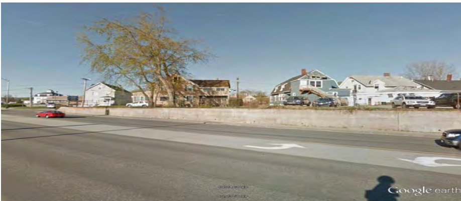
Center Street, West side between Grove and Vernon – Concrete wall constructed by the City in 1957.
