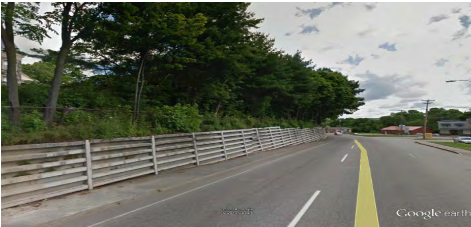
Minot Avenue Rotary – Metal bin wall constructed in 1957. A Maine DOT and City project will be replacing the bin wall in 2014.
